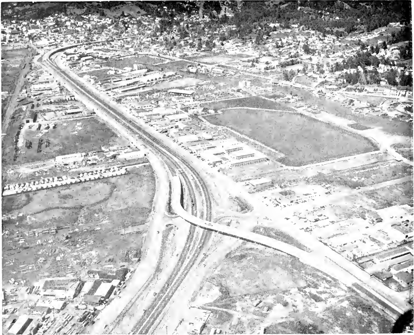
Redwood Highway looking north toward San Rafael from vicinity of California Park Wye
